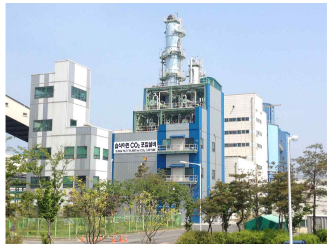
Fig. 4. Photos of 10 MW CO 2 capture plant located at Boryeong thermal power station.
