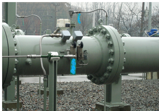
Fig. 1. Example of branch lines attached aboveground high pressure natural gas pipeline in a regulating station.
